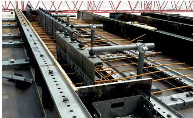
Easy Form in combination with UAR adapter
