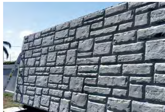
Noise barriers, USA
