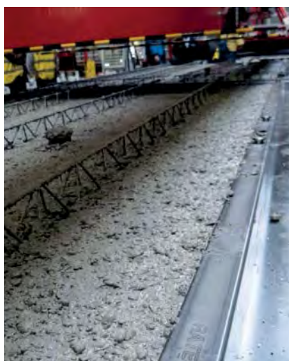
Girder slab production
