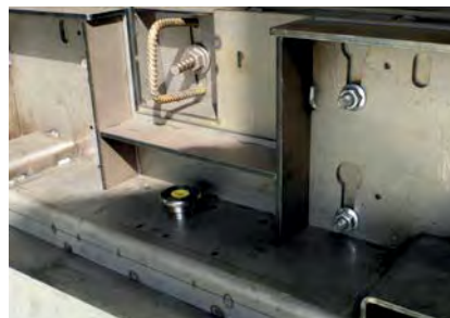
SAS-MF with extension modules for continuous reinforcement
