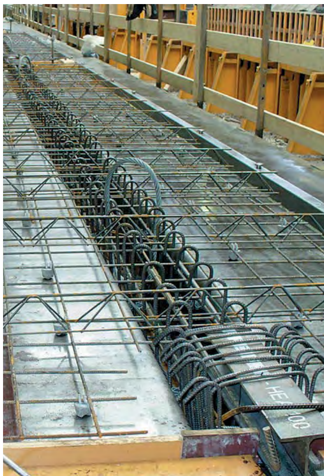
TT slabs production
