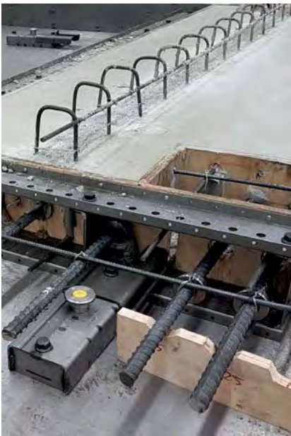
Easy Form with continuous reinforcement
