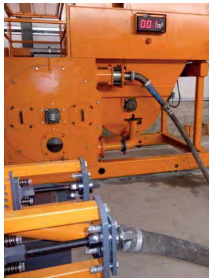
Concrete filling connection UCI Square
