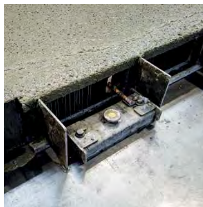
MST after concrete pouring
