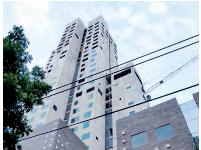
Facade elements, Indonesia
