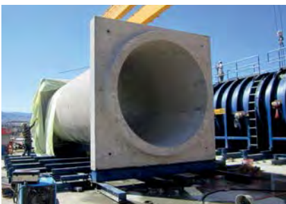
Shaft element pumped with UPP
