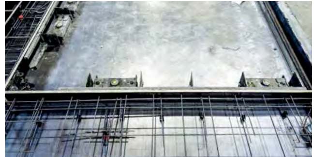
Recess with MST and wooden window corner
