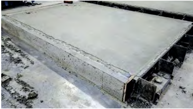
Recess with MST and wooden window corner
