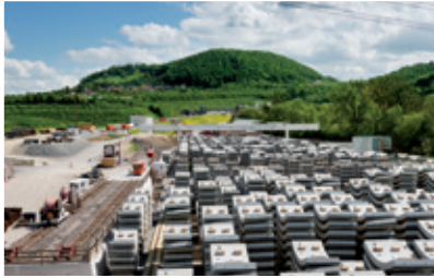
Bossler Tunnel Stuttgart / Ulm, Germany
